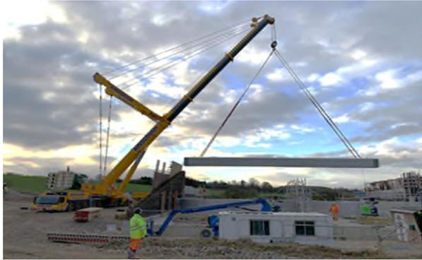
River Ash bridge beams being lifted into place
